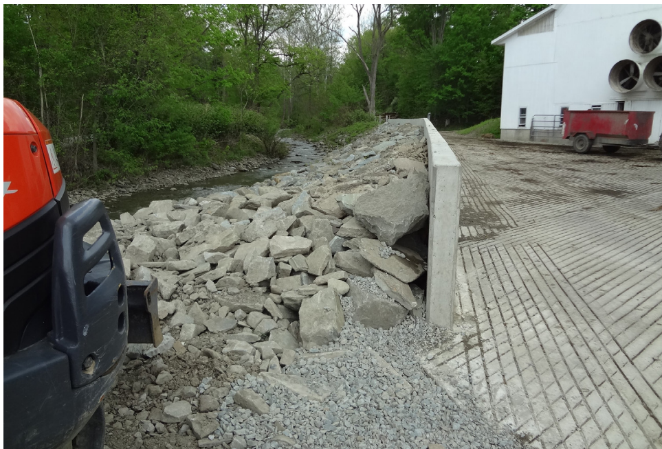
Protective streambank riprap to protect against erosion.
